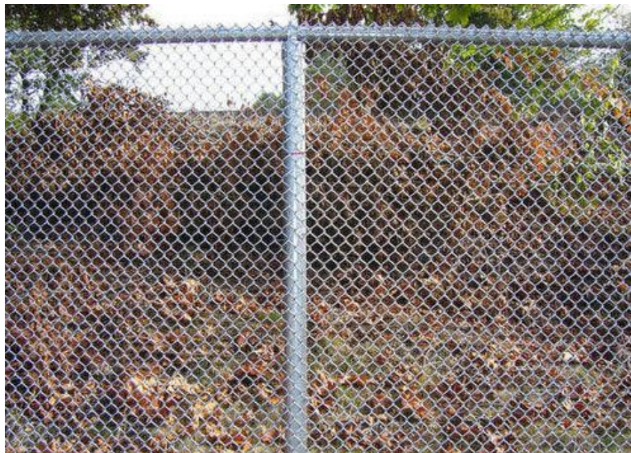
8' tall, "no-climb" chain link fence
